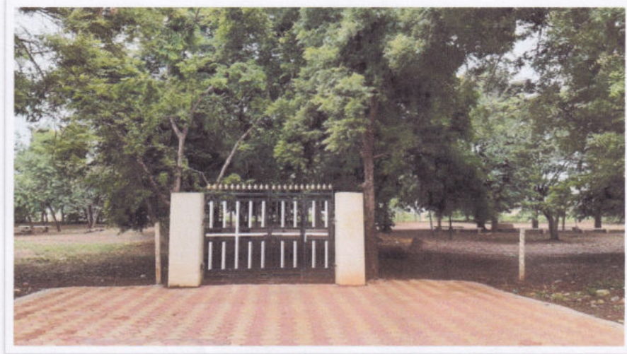
Pic -6 Garden Entrance
